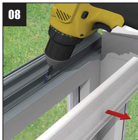
08 Drill a 5mm pilot hole in the head of the frame, fasten down using 4.8 x 32mm screws (not supplied) at 450mm centres. Refit internal claddings. If fastening up through the frames into the eaves beam use 4.8 x 55mm screws.
