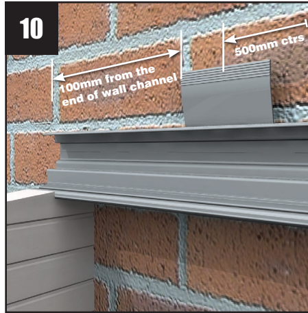
10 Offer the wallplate up to the wall and position it so that the top surface of the bolt slot is level with the top of the firrings.
