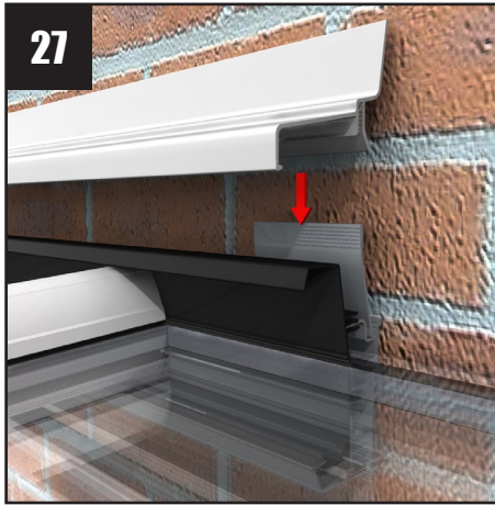
27 Cut the pvc wall plate top capping to the overall width of the conservatory (externally) and notch over the top of the lean-to cloaking trim at each end. Push fit the wall plate top capping.
