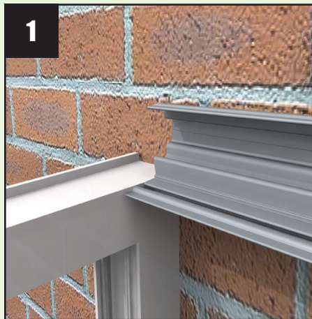
1 Offer the wallplate up to the wall and position it so that the top surface of the bolt slot is level with the top of the side frames.
